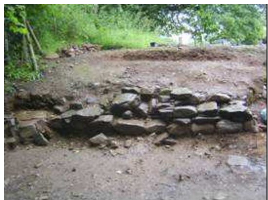
The “yard area” retaining wall
